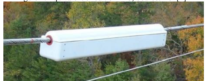
Figure 5: Series FACT device clipped on Transmission Line Source: Ref [2]
